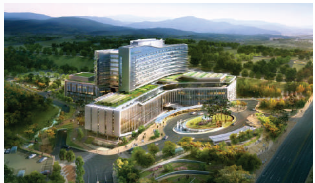
GyungSang Univ. Hospital 300RT 2units
