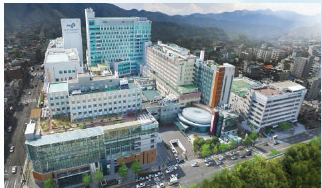
Busan University Hospital 320RT 4units
