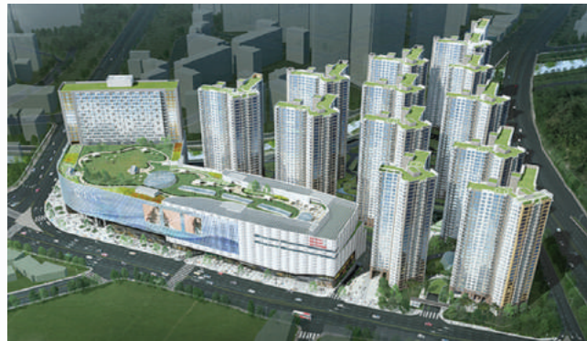
Lotte Mall 1050RT 3units, 600RT 1unit, 155RT 2units
