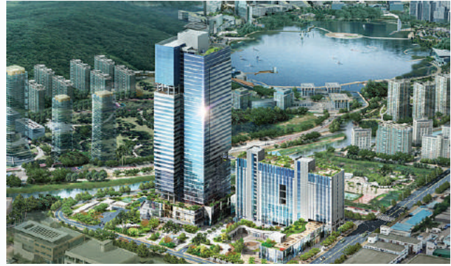
IT Valley 825RT 5units, 270RT 3units
