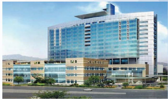
Hanlim University Hospital 900RT 2units
