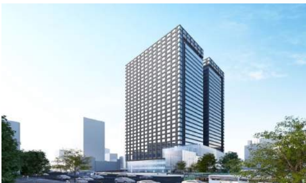
Namdaemun office building 560RT 2 units
