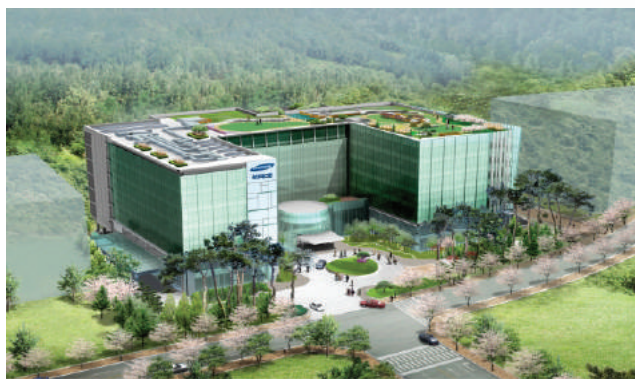
Hanwha Techwin 675RT 3units
