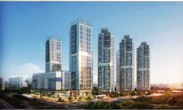
Complex Building 470RT 2units, 340RT 4units
