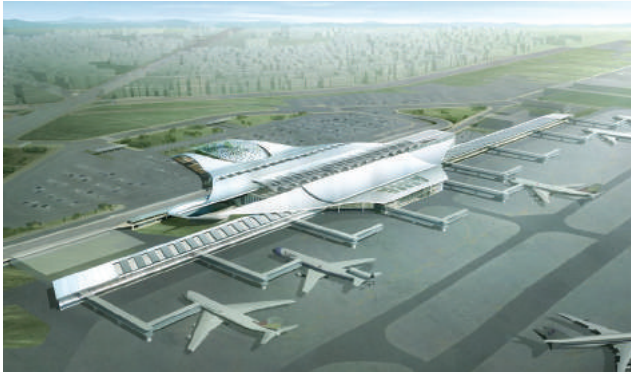
Gimpo Airport 700RT 12units
