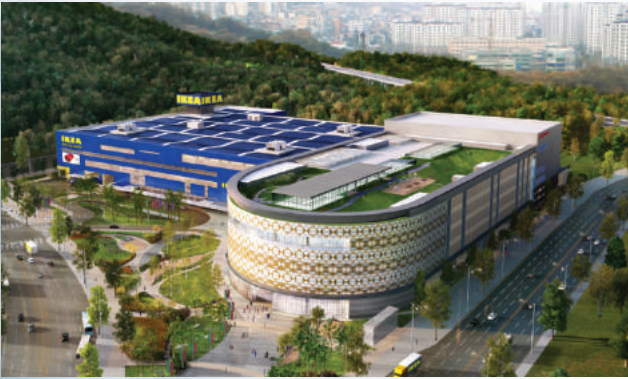
Lotte Outlet 600RT 7units, 135RT 2units
